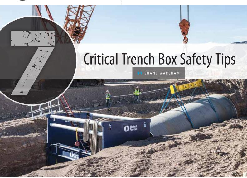
If working adjacent to a critical structure (roadway, railroad track, or building) and it is important to eliminate soil movement from under that structure, shoring may be a better option.
