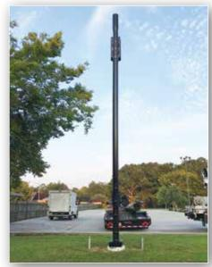
This Small Cell Services tower augments existing cellular coverage and converts it to 5G allowing for 5G coverage to reach more communities without a complete overhaul of legacy cellular infrastructure.
